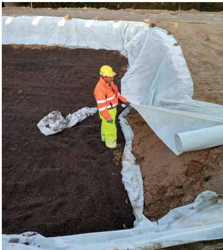
Polypropylene Geotextile installation (250 gr/).
