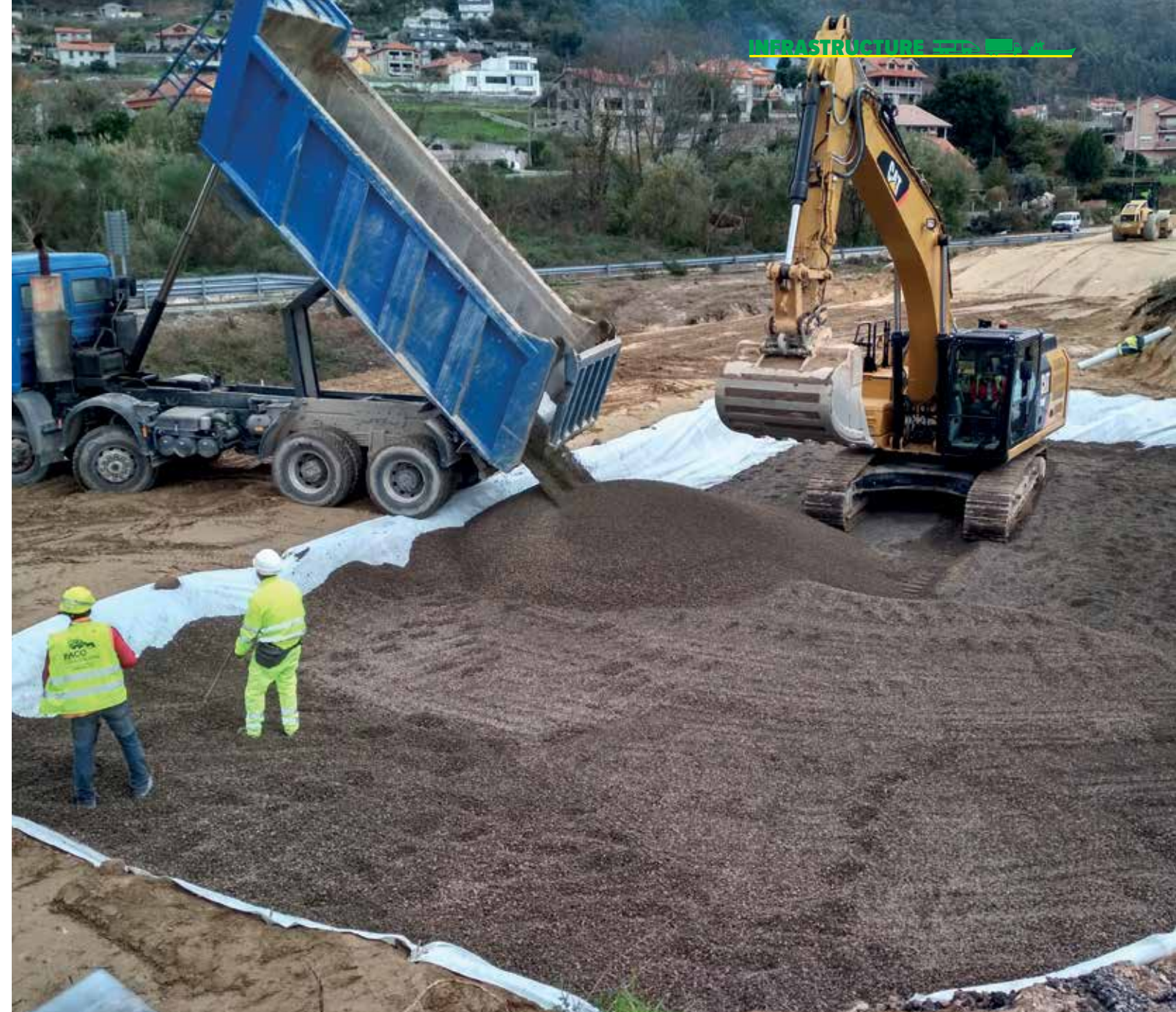
Installation of Arlita® on the structure.
