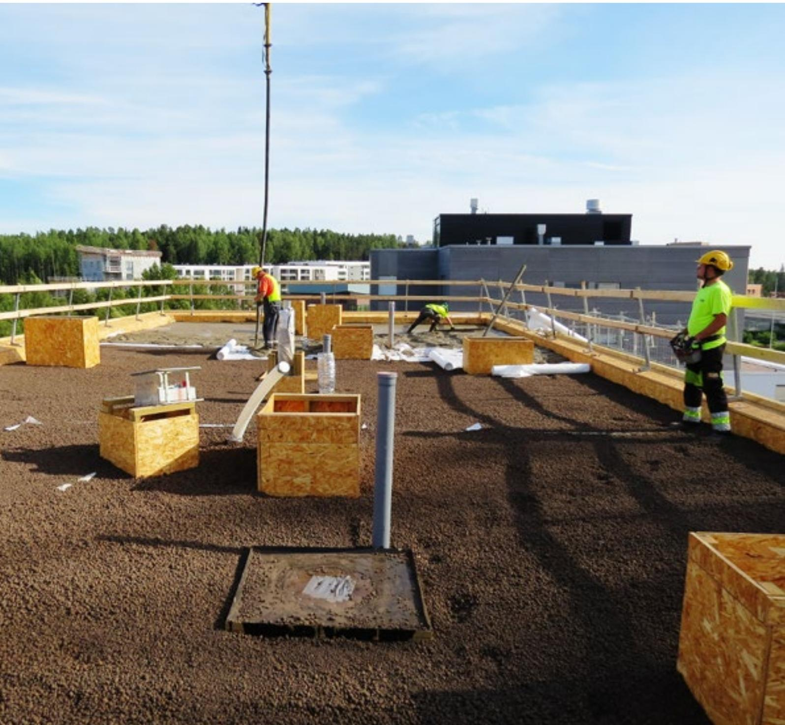
**Competent professionals** quickly cast and knead the thin concrete slab that will become a base for the final waterproofing.
