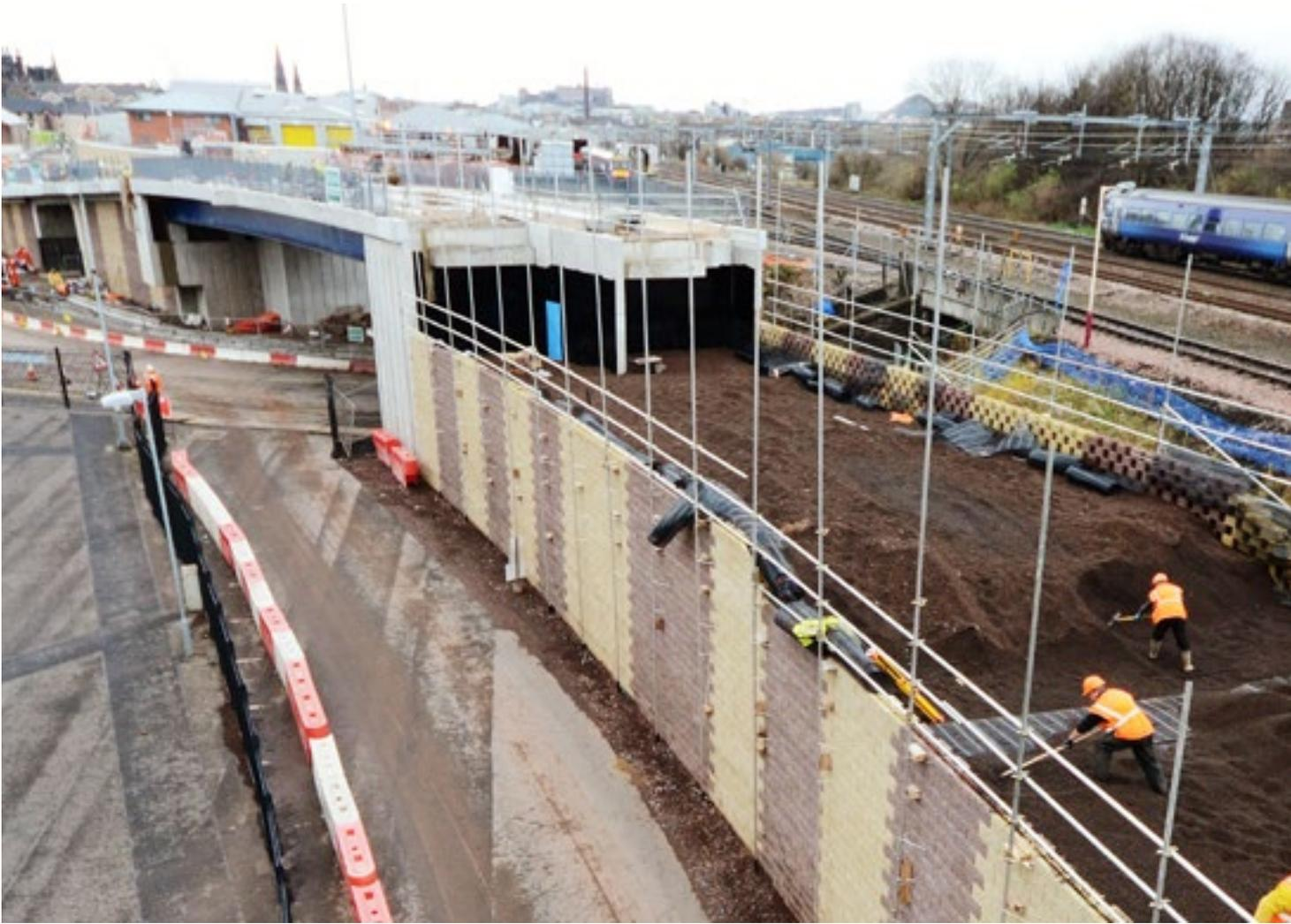
To create a stable and high raised tramway system in Edinburgh, the Murrayfield tram stop was built on Leca lightweight aggregate.
