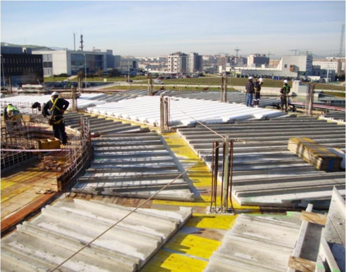
Building a circular structure represents a challenge for prefabricated concrete elements. A new and innovative solution was needed to build the new headquarters for Gamesa in Pamplona in Spain.
