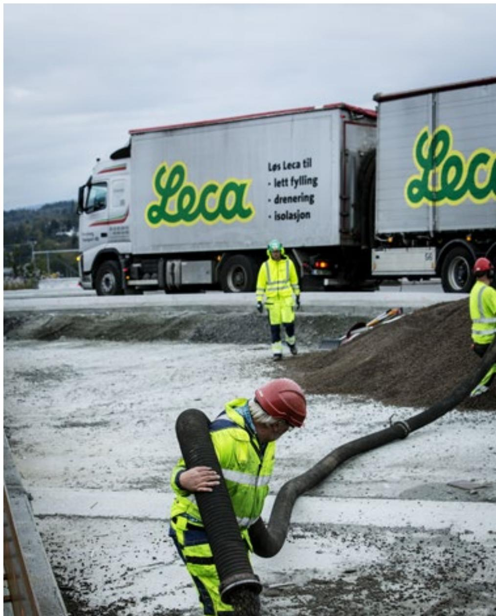
**To reduce the weight** of the roundabout on Highway 4 in Norway, the developer chose Leca aggregates as filling for the plant beds. The aggregates were blown in place through a series of hoses.
