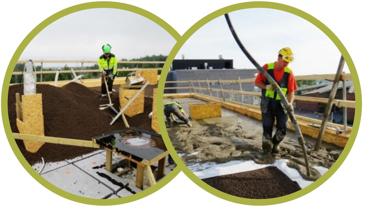
The 220 apartments under construction in Saunalahti in Finland will have a ventilated structural Leca aggregate roof.
