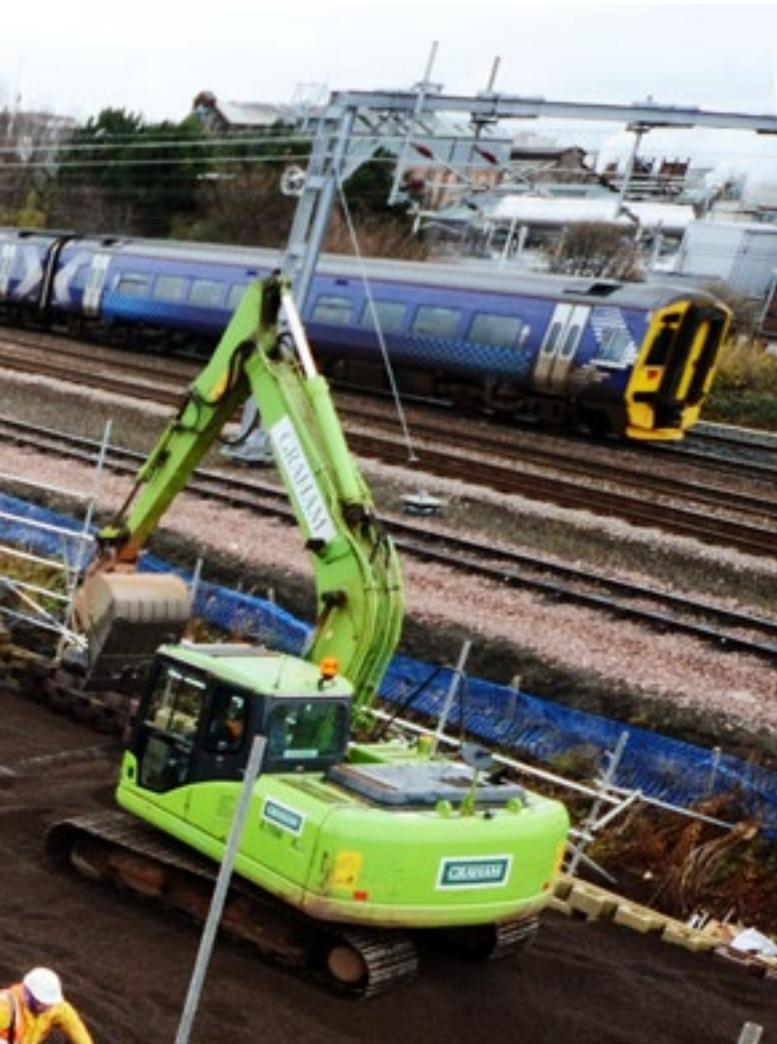
**Bearing and stability** concerns made Leca aggregates to be the perfect material for infill when constructing the Murrayfield tram stop in Edinburgh.
